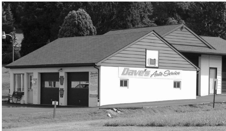
Shown is Dave's Auto Service garage.
