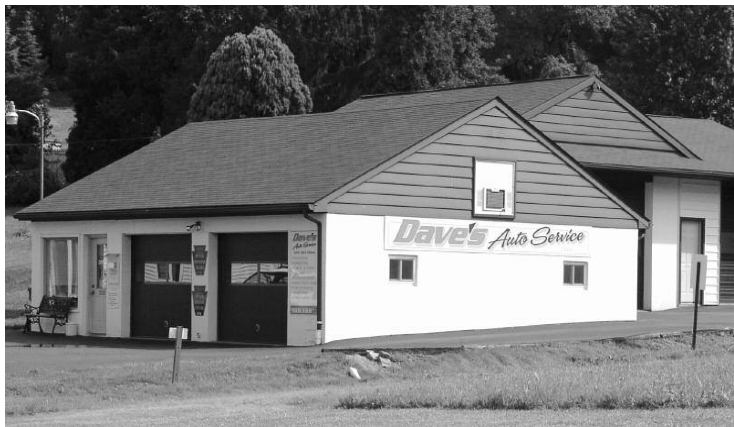
Shown is Dave's Auto Service garage.
