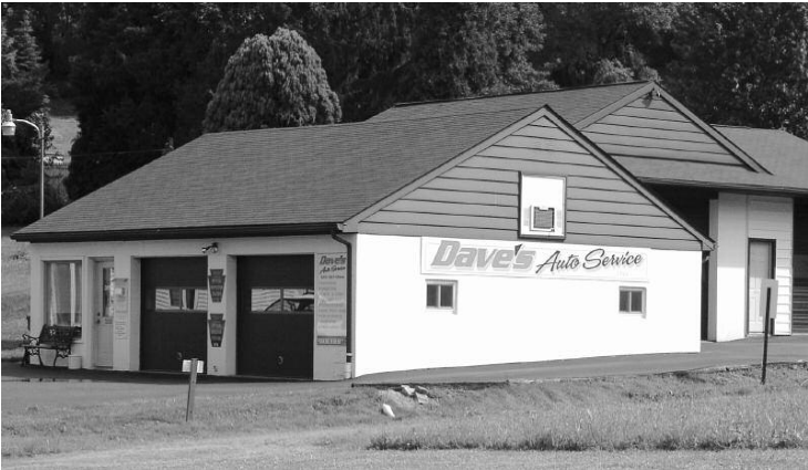
Shown is Dave's Auto Service garage.
