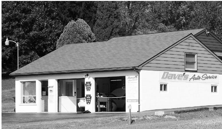
Shown is Dave's Auto Service garage.
