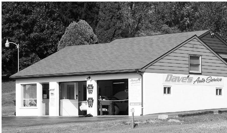
Shown is Dave's Auto Service garage.
