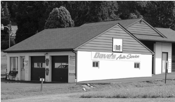
Shown is Dave's Auto Service garage.
